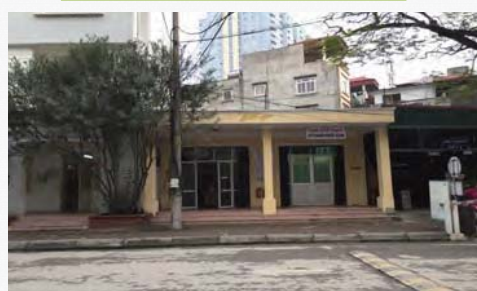
Setting up centralized linen storage
